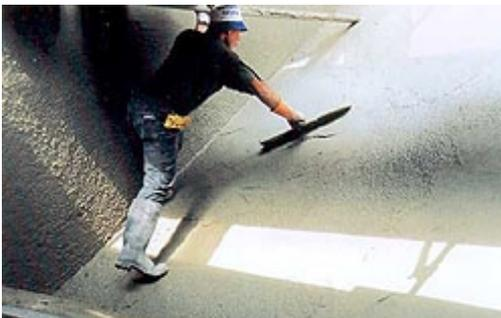
**Levelling the freshly applied mortar coating**
